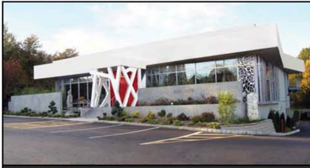
EIFS and poured concrete exterior finishes are offset by a distinctive portal designed to have the look of a Corian finish.
