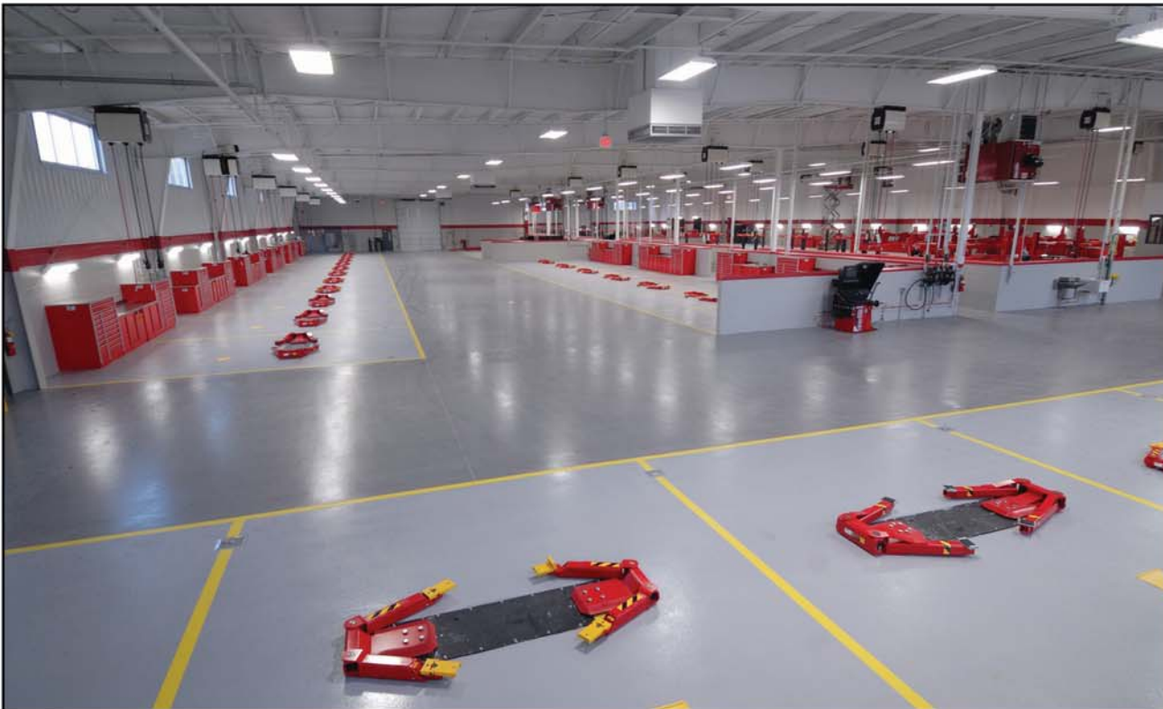
80,000 square feet of shop areas were constructed using pre-engineered steel to enable an 80' clear span roof system.
