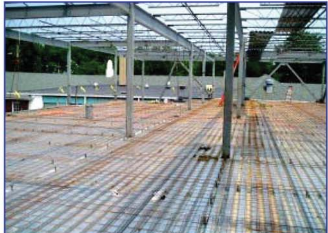
Second level. Floor deck (below) and open bar joist (above).
