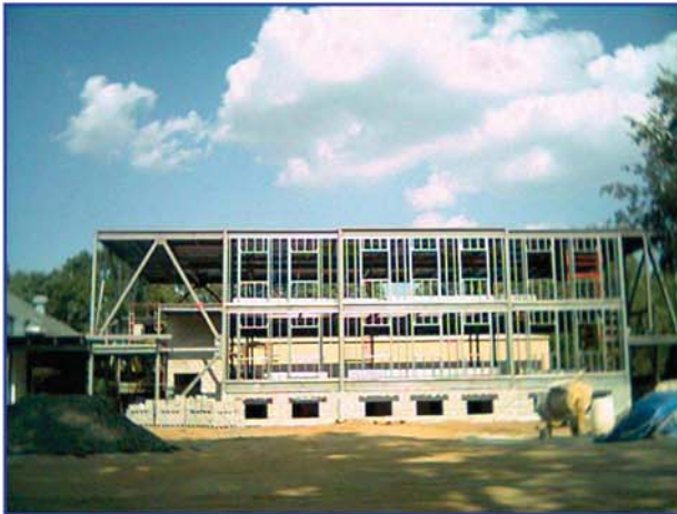
Front of building showing structural steel and light gage framing.
