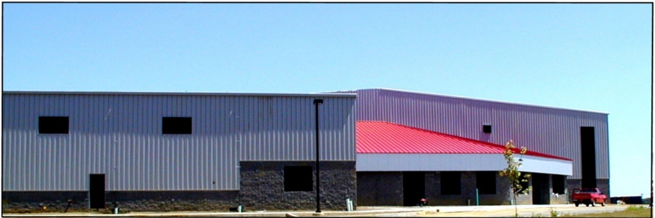
Right wing houses soccer arena and roller rink at 192' x 90' each. Left wing for future Gold's Gym at 22,000 SF. Note: Progress photo, three months prior to completion.
