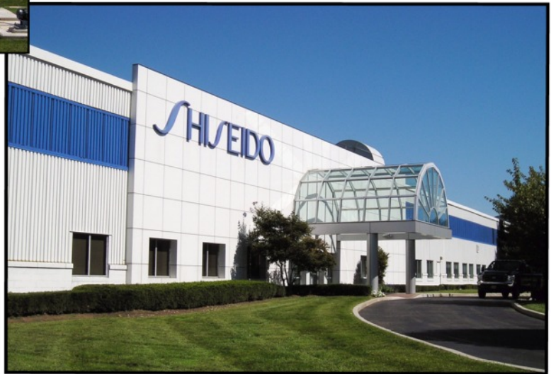
An exterior view of the existing building and main entry
