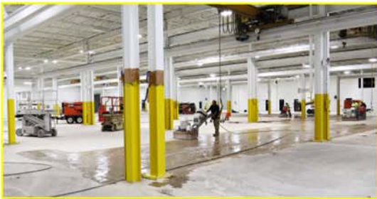
Polishing concrete
