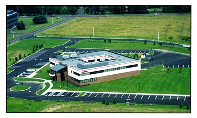
The Land Instruments building is situated on a 5-acre site. The two-story structural steel building has walls consisting of brick and dryvit. The clear-story front foyer has a barrel vault standing seam roof and interior brick veneer walls.
