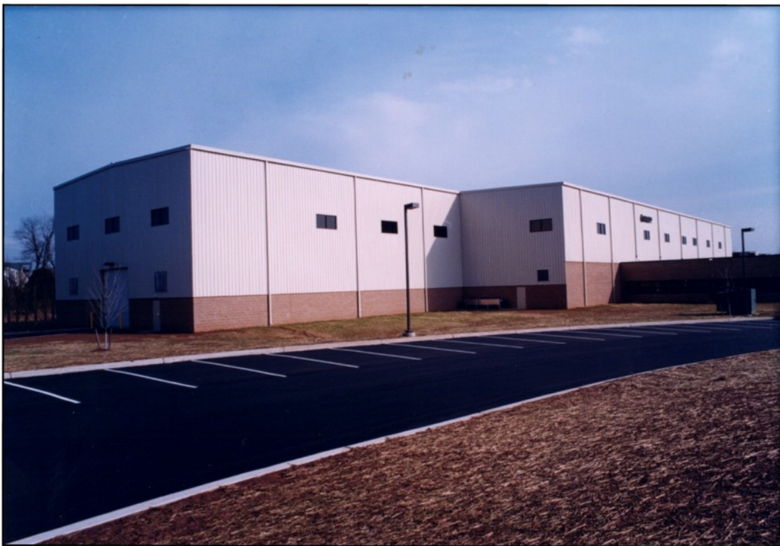
Both sections completed
