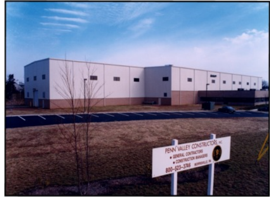
Addition nearing completion in 1999
