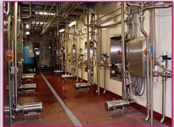
Silo Tank Hall
