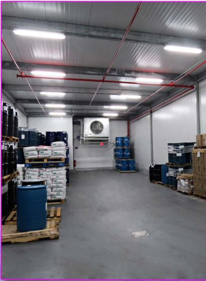
Above: Cold storage warehouse
