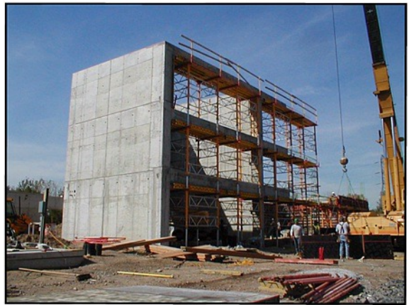
The manufacturing building is an H-3 occupancy constructed with reinforced concrete designed to meet the damage limiting requirements of NFPA 68.
