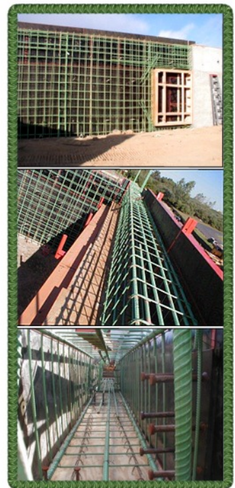
Reinforcing steel bars with an epoxy coating are used to provide "DLC".
