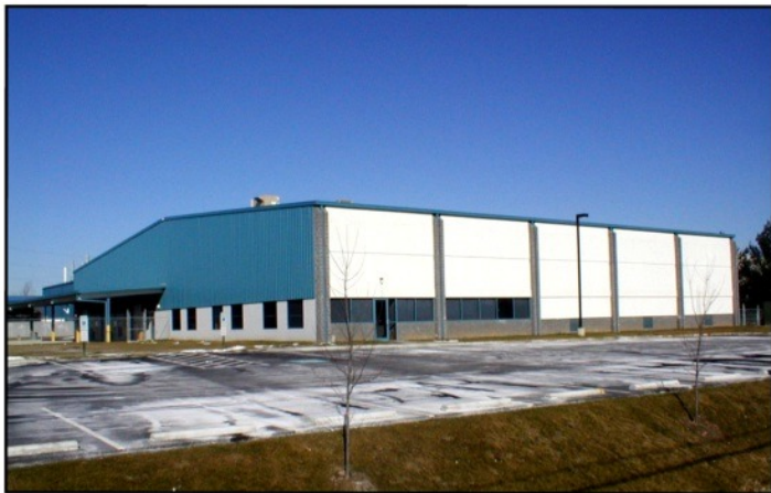
Gelest's Office-Warehouse is a pre-engineered building featuring Dryvit, metal siding, rockface and painted block. Vapor detection and emergency ventilation are included to meet the requirements of NFPA 69.
