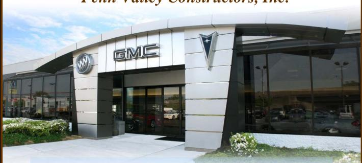
Renovations to Faulkner GMC included new ceilings, floor tile and wallcoverings for the showroom and office areas. A metal paneled entry tower was constructed following a new Retail Image Program.
